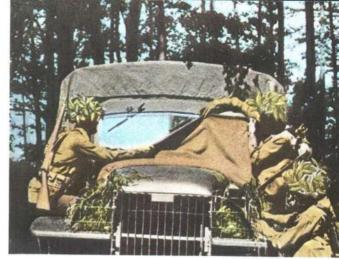
FIGURE 21. — The wise driver makes his own slip-on covers for headlights, windshields, and other reflecting surfaces. He keeps them covered at all times, if possible. They may be made of pieces of burlap, osnaburg, or salvage.
