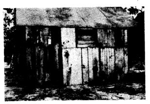
FIGURE 70 ① and ②.—Two examples of deception in hiding supplies. Boxes have been stacked in a mass to resemble buildings. Simple frame roofs complete the disguise. Such roofs are designed to resemble type of buildings found in the area.
