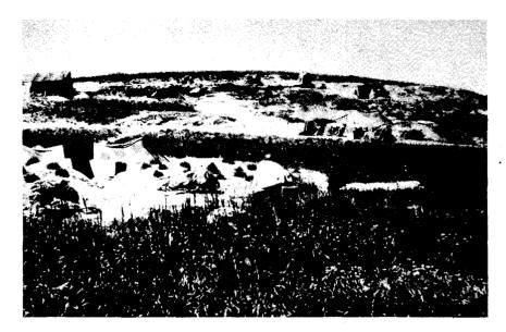
FIGURE 19.—Bivouac in scarred grassy area in a theater of operations. Tents are dug in as much as possible, painted in disruptive patterns, dispersed, and made to look like hummocks. Tufts of vegetation have been transplanted in the area to give texture to it.
