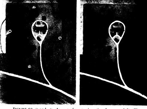
FIGURE 50 ① and ②.—Layout of protective wire shown on left will invariably attract attention to a command post it surrounds. Wire must not be laid across fields in lines contrary to normal ground pattern, but along existing lines of cultivation and along natural boundaries, as shown at right.
