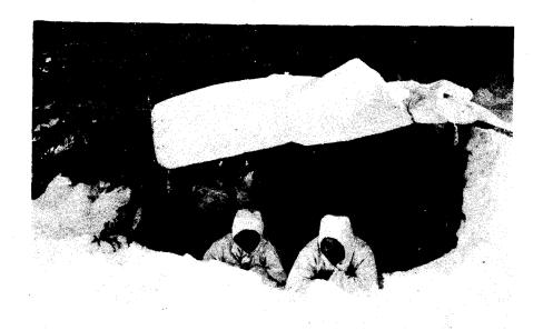
FIGURE 24.—Shelter halves painted white and used in conjunction with post supports and natural materials to provide shelter and concealment. Trees and branches placed around the outside of the structure aid in camouflage. Whenever possible pile snow irregularly around tents and other objects to aid in blending.
