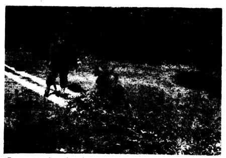
FIGURE 32.—Sometimes it is possible to tone down short stretches of newly made road by brushing leaves or placing brush upright over them. Complete concealment is extremely difficult, however, and only aerial observation can give an accurate check on the success of the work.
