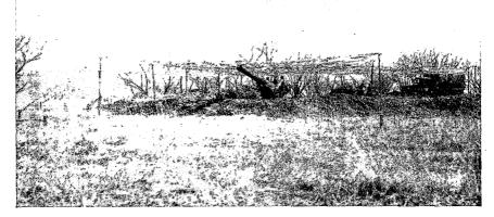
FIGURE 53.—This photograph illustrates a dug-in 155-mm gun position at which flat-top does not cover all the spoil. Supplementary camouflage is necessary to conceal such a position. Flat-top is extended around edges, either with additional nets or with garlands.
