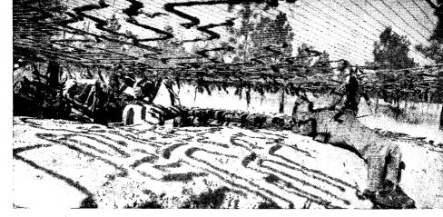
FIGURE 50.—Areas between nets *must* be garnished with additional burlap strips or textured patches.
