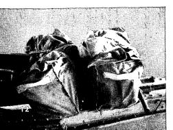
4). — Bags attached to 155-mm howitzer M1817A4 or M1918A3. Straps cross on top and loop around side rods of loading barrow. These are released by removing fastening pins of loading barrow.
